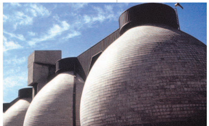
Egg-shaped Digestors
